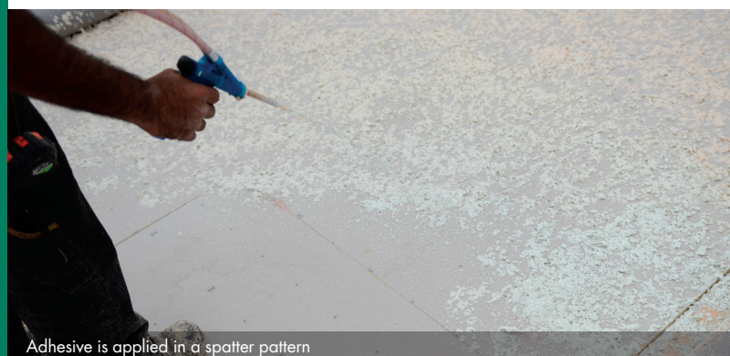
Adhesive is applied in a spatter pattern
