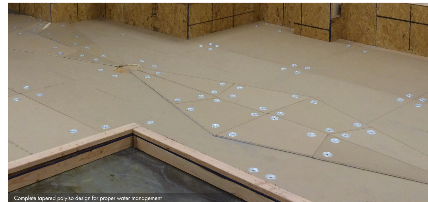
Complete tapered polyiso design for proper water management
